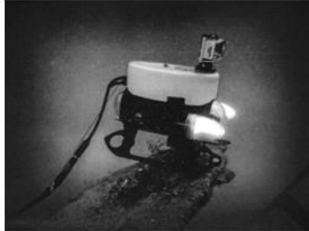
Figure 7.1 Underwater inspection using ROV. Source: Diving Status (permission to use image granted by copyright holder)
