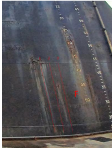
Figure 72: Floating Dock Lateral Surface and Inspection lines
