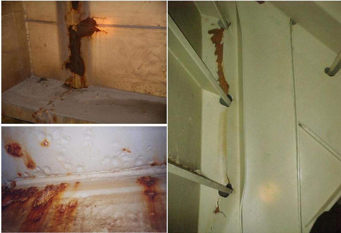
Figure 1: Examples of coating breakdown and corrosion (CBC) affecting ship surfaces.
